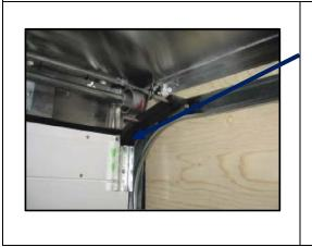
For most doors the top of the silver bracket will be  $+ / - \frac{1}{4}$ " from the top of the door. The top roller brackets should be secure and parallel with the tracks, in from the panel edge by  $\frac{1}{4}$ ".
