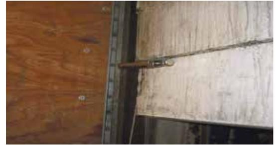
**Step 7** If the bottom panel is to be replaced, disconnect the cables from the u bolts and remove the vice grips holding the bottom panel. If the bottom panel is not being replaced, leave the vice grips attached
