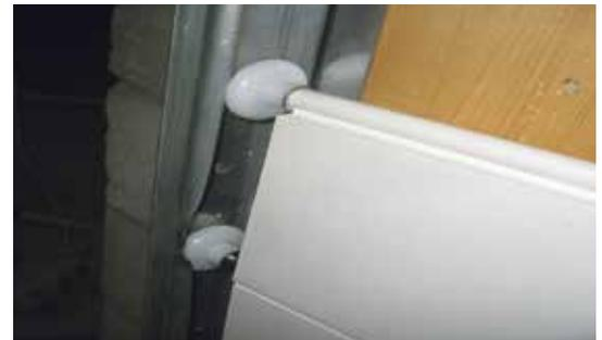
**Step 14** Hammer the bent out track back to its original shape
