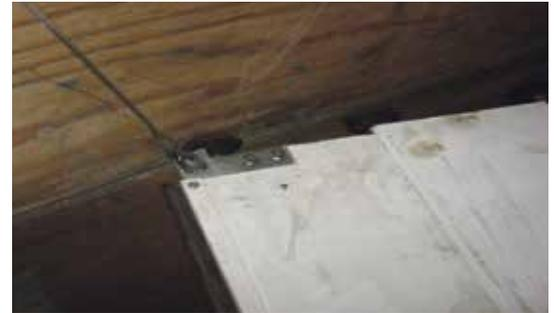
**Step 12** Install one end of the door into the tracks and begin to rotate the panels back toward the door opening.
