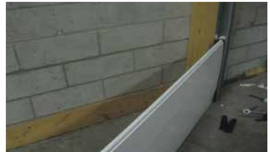
**Step 13** Starting with the bottom rollers first, install the rollers through the bent out section of track.
