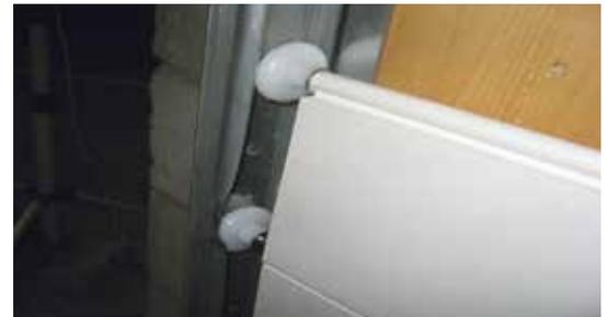
**Step 9** Once the rollers are out of the tracks, on the one side, remove the damaged panels.
